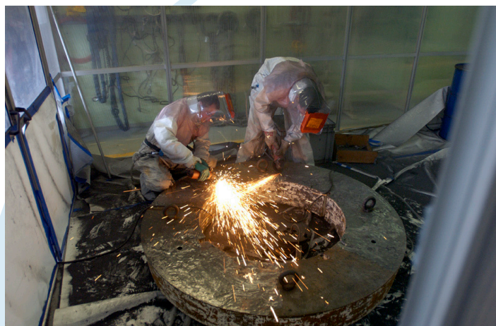
Dismantling of Belgian Reactor 3 (BR3) in a ventilated booth.
