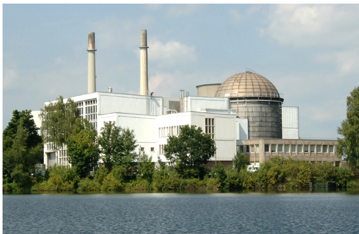
Outside view of Belgian Reactor 3 (BR3).
