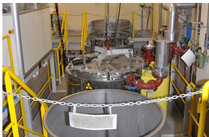
Chemical decontamination of metal parts (MEDOC).
