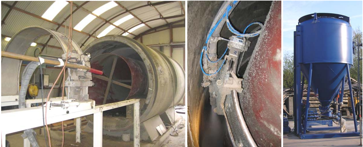
Dry grouting tests: grouting vehicle (left and centre) and dry-gun machine (right).
