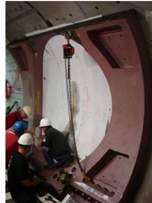
Reinforcement structure: milling of the structure as a whole (left) and assembly underground (right)
