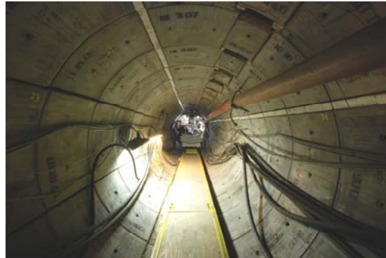
The left picture shows the tunnelling equipment as it is positioned into the reinforcement structure: the road header (painted red) is visible at the front of the tunnelling shield; Boom Clay is visible in the opening of the reinforcement structure. The right picture shows a view of the PRACLAY gallery under construction. The concrete wedge-block lining is visible, as are the dilation joints made of compressible stainless steel foam (painted white).
