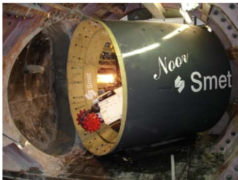
The left picture shows the tunnelling equipment as it is positioned into the reinforcement structure: the road header (painted red) is visible at the front of the tunnelling shield; Boom Clay is visible in the opening of the reinforcement structure. The right picture shows a view of the PRACLAY gallery under construction. The concrete wedge-block lining is visible, as are the dilation joints made of compressible stainless steel foam (painted white).
